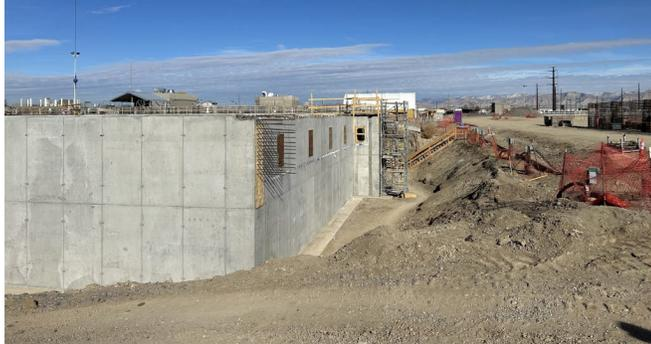
As part of the expansion, Xypex Admix C-500 was incorporated at the time of batching into the concrete used for the facility's new water-holding structures. By integrating Xypex directly into the mix, the need for traditional surface-applied waterproofing methods was eliminated, resulting in significant cost savings and long-term durability.
